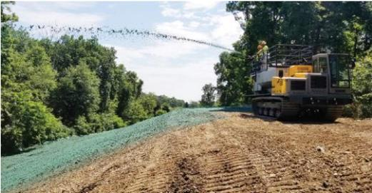
Photo Caption 3: Terramac with hydroseeding unit spraying cover with grass seed.
